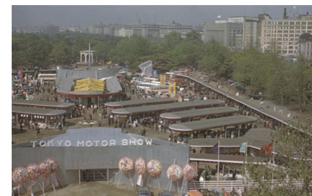
The 1st Tokyo Motor Show, Hibiya Park, 1954
