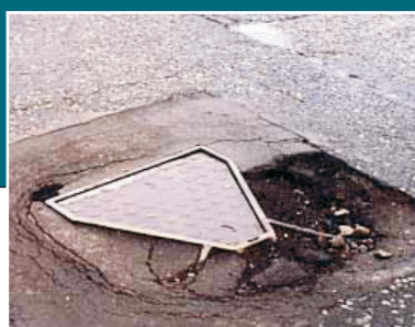
Drains (covers) can be a problem for PTWs, because of the loss of surface grip (source: ITC, Bulgaria)
